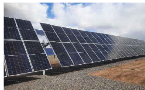
TYPICAL TRACKER - SINGLE AXIS TRACKER - TWO MODULE IN PORTRAIT
